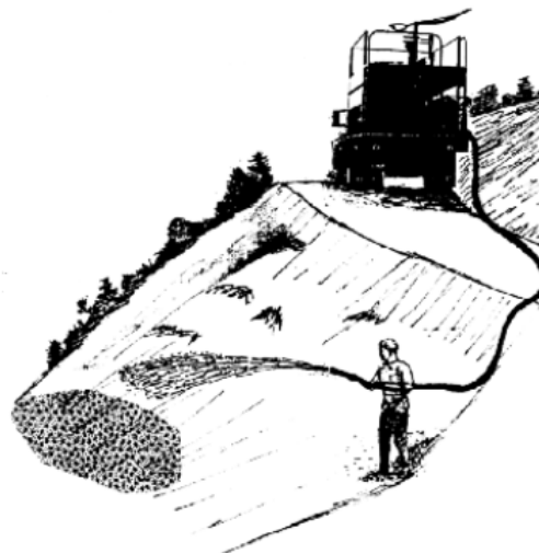
Figure 34: Hydroseeder attached to truck
